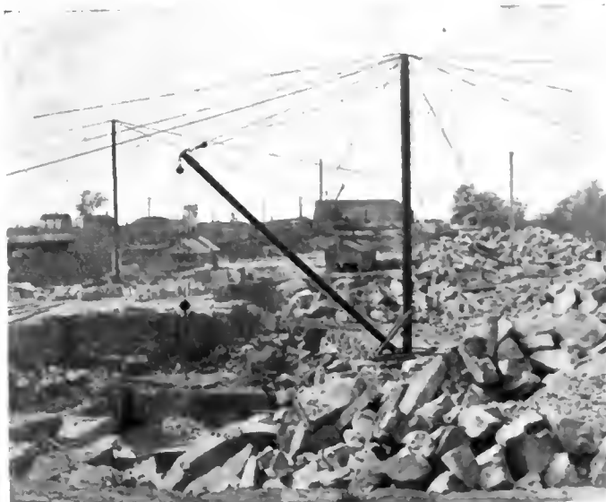
General view of Queenston Company's quarry at St. David's, June 1, 1916.
